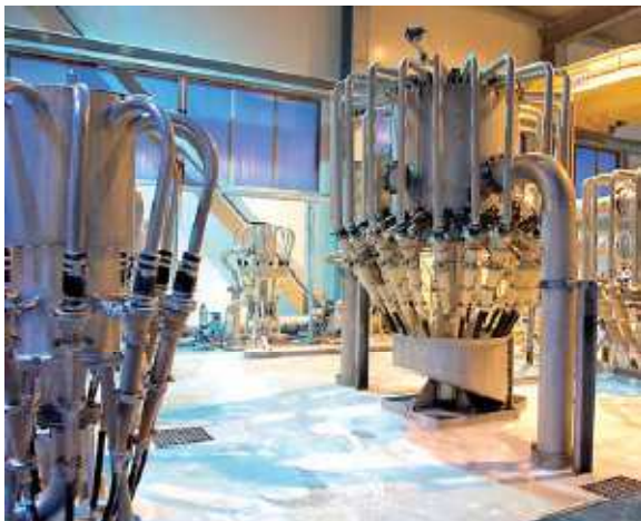
Figure 4. Fluidized bed reactor for cadmium removal
