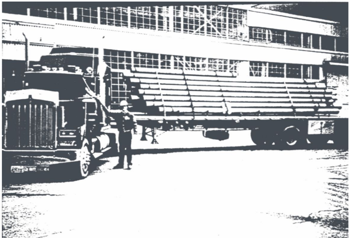
Fig. 42 - Beta C downhole piping
